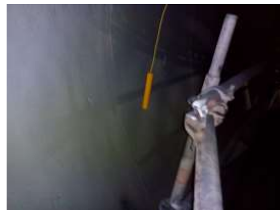
Figure 3. Permanent reference cell #3 near the wall of the bowl area inside the elevated water tank prior to commissioning.
